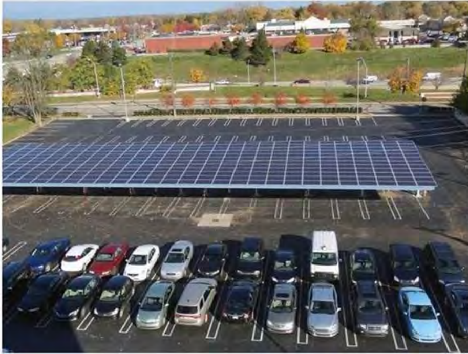
Figure 7.7-14: Solar panels at 1-800-LAW FIRM. 61
