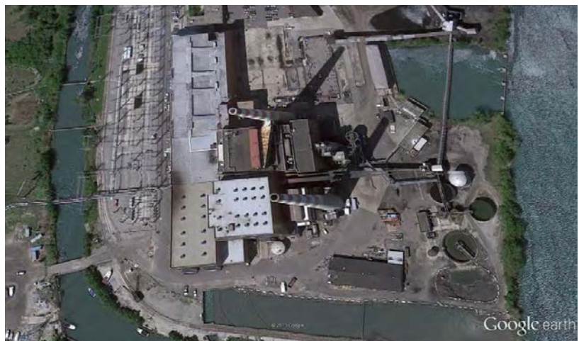
FIGURE 1. Example of point source: Trenton Channel Power Plant located at 4695 Jefferson Ave., W Trenton. This is a major source (greater than 100 tons/year) of SO 2 , NO x and PM 2.5. From RACT Analysis SIP and Google Earth.
