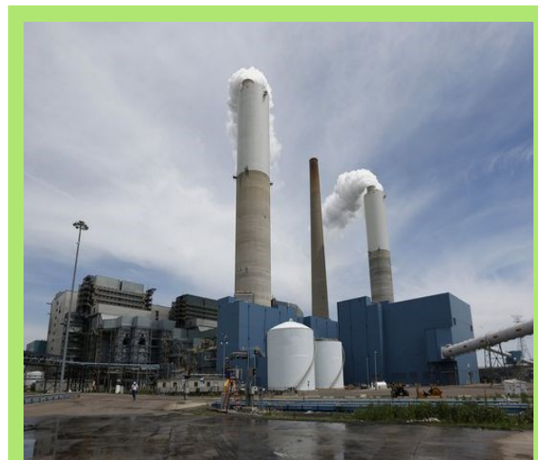
DTE Energy's Monroe Power Plant (Photo: Bloomberg)
