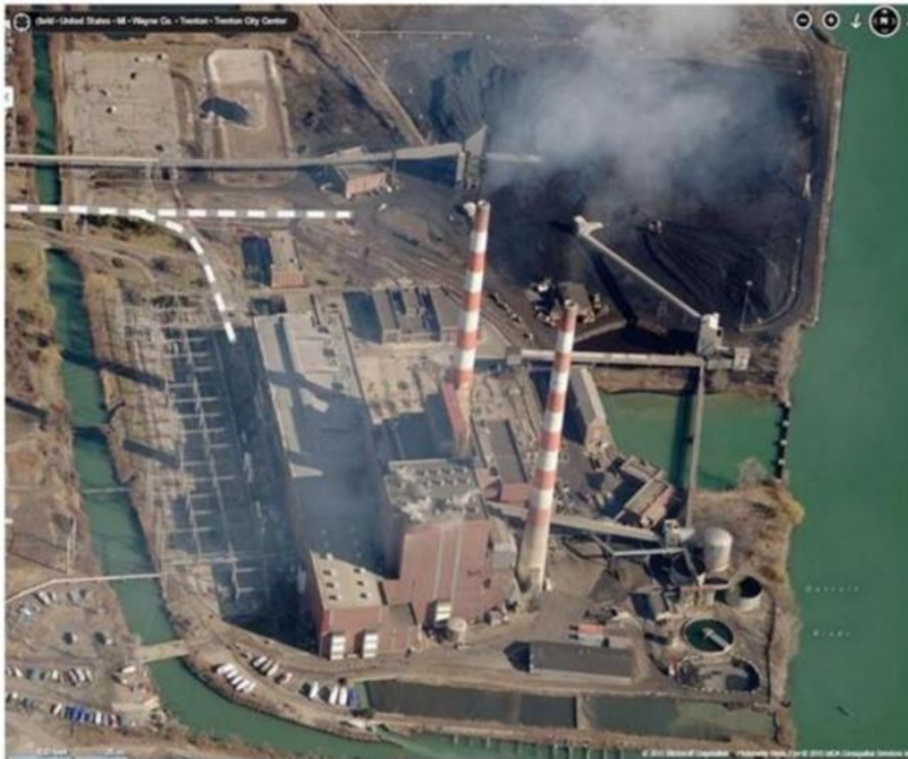
Figure 5-1. Aerial photo of the Trenton Channel power plant, which can burn coal, natural gas, fuel oil and residual paint solids, is an example of a major point source in southwest Detroit. Each stack is over 560 feet tall. Photo from Google Maps.
