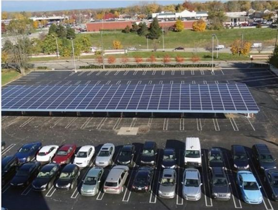
Figure 7.7-14: Solar panels at 1-800-LAW FIRM. 61
