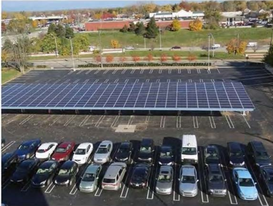
Figure 7.7-14: Solar panels at 1-800-LAW FIRM. 61
